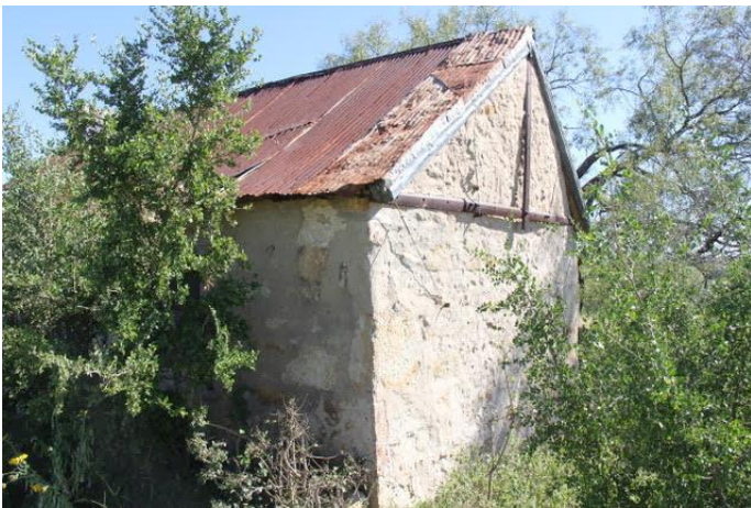
Beauregard Ranch out-building. Example of white sandstone. Photo by Allen Kosub. Located on private property. Photo taken with permission of the property owners.
