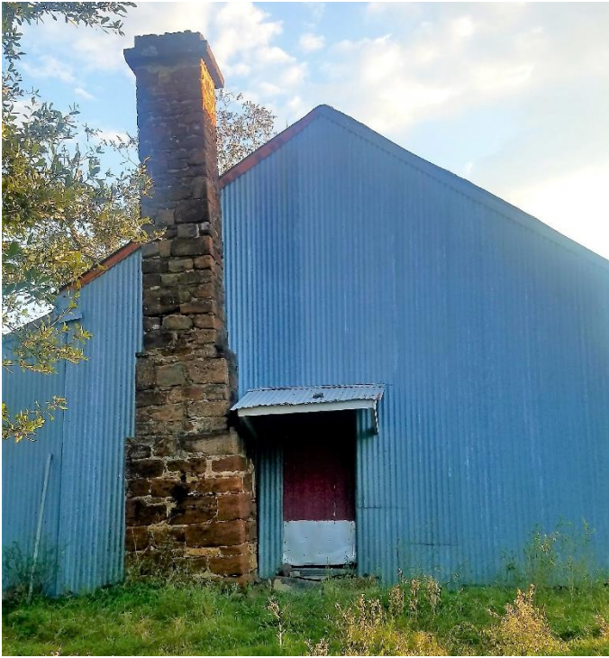
Red sandstone rock chimney on the Suhre Store built in the 1800s in La Vernia. Located on private property. Photo courtesy of the La Vernia Historical Assn.
