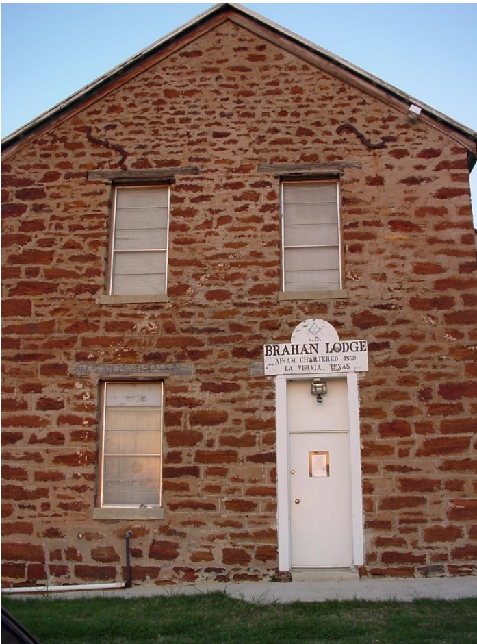
Brahan Masonic Lodge, La Vernia. An example of red sandstone. Photo courtesy of the La Vernia Historical Association.
